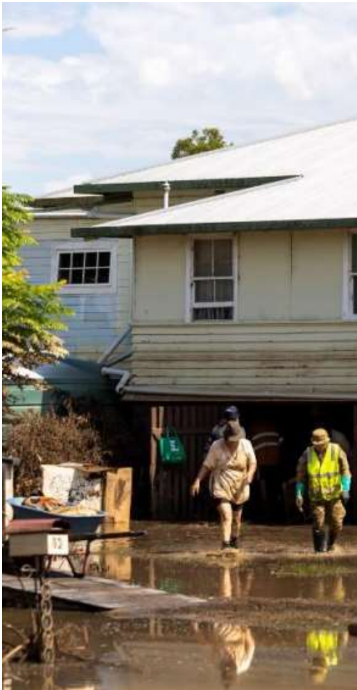
Flood Damage. Source: Australian Army Twitter
